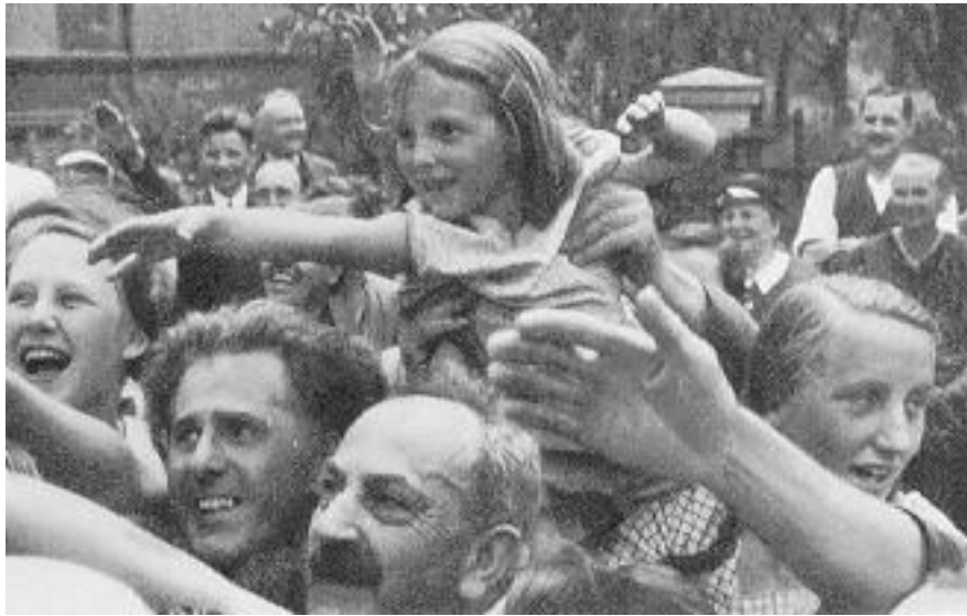
The Leader leaves the construction site of the House Of German Art.
