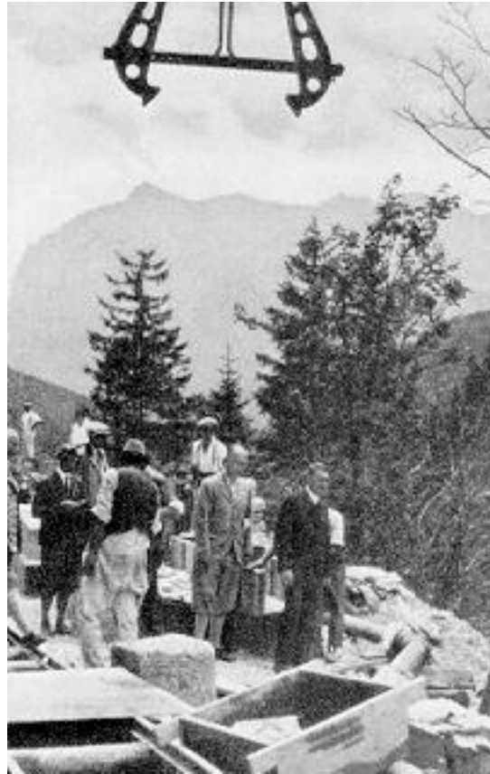
The Leader's interest in road construction: inspection of the Alpine Road.
