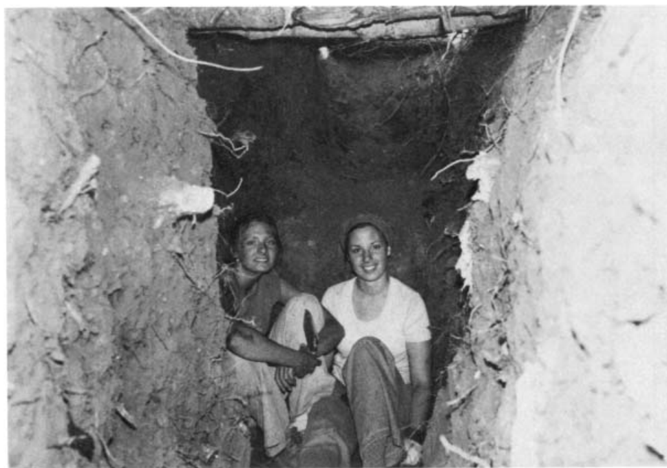
Fig. 5.2. Two non-athletic college girls who completed a 4-person Pole-Covered Trench Shelter in 35½ hours, despite tree roots.
