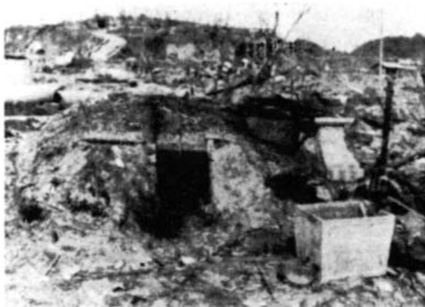
Fig. 1.5. Undamaged earth-covered family shelter in Nagasaki.
