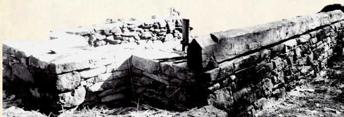
Figure 22. Stone foundation & V-shaped log
