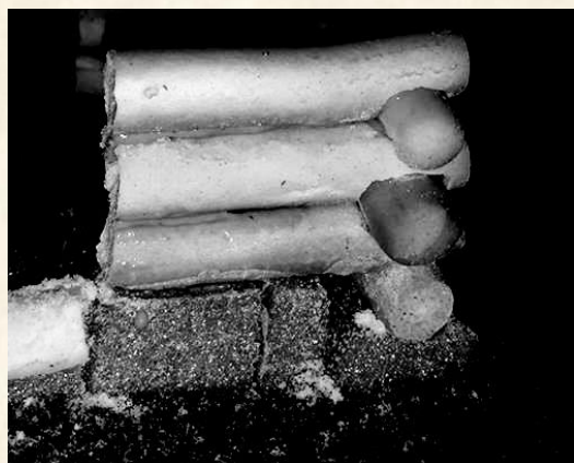
Figure 20. Log notching on round-shaped logs
