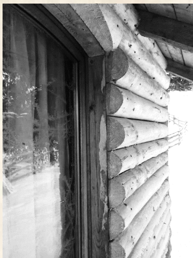
Figure 25. Window framing
