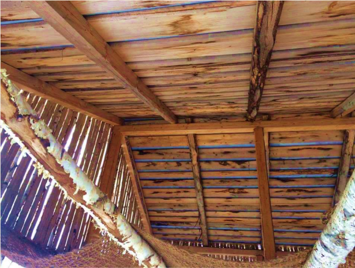
Figure 34. Roof boards for coverage
