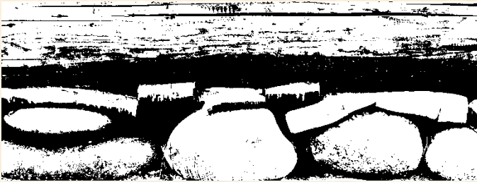
Figure 18. Stone foundation, tar oakum & moss with sill
