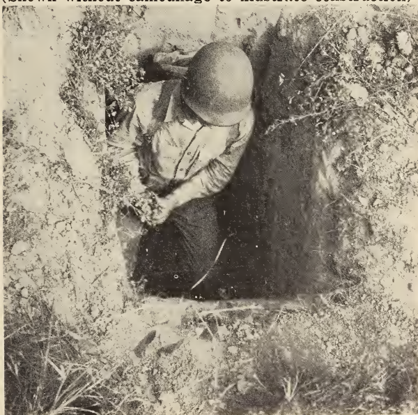
FIGURE 8 Rectangular type foxhole (Shown without camouflage to illustrate construction)
