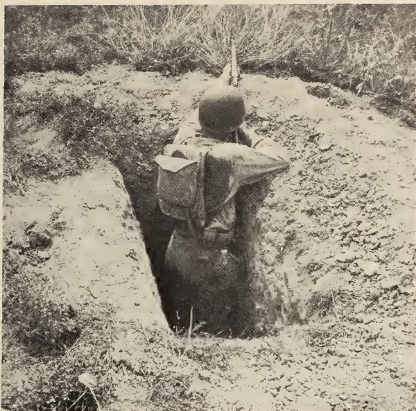
FIGURE 8 Rectangular type foxhole (Shown without camouflage to illustrate construction)
